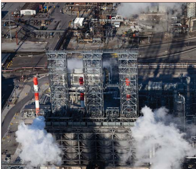
BP petcoke processing plant in Whiting, Indiana Photo: Terry Evans
